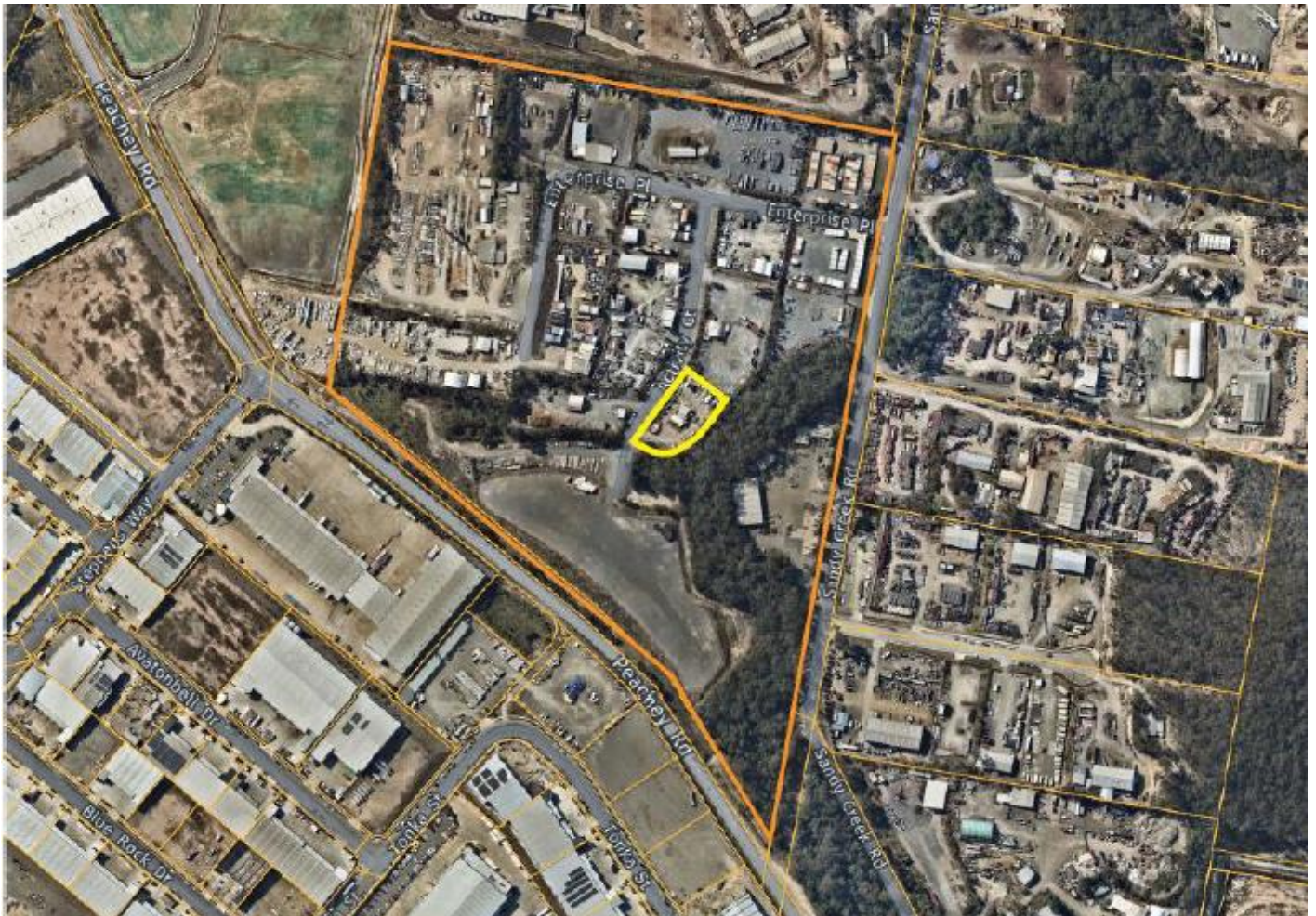
Figure 1: Aerial view of Lot 98 on Plan SP320866, identified in orange. This activity is operated at 3 Activity Court, Yatala, depicted as the part of Lot 98 identified in yellow.
